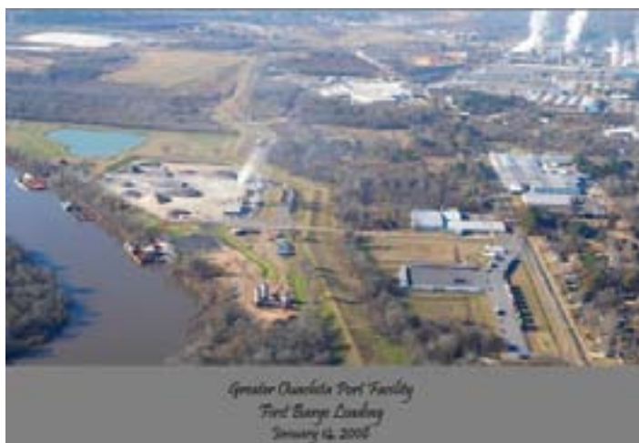
Greater Ouachita Port Facility, West Monroe, LA
